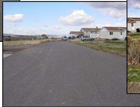
Street Looking West
