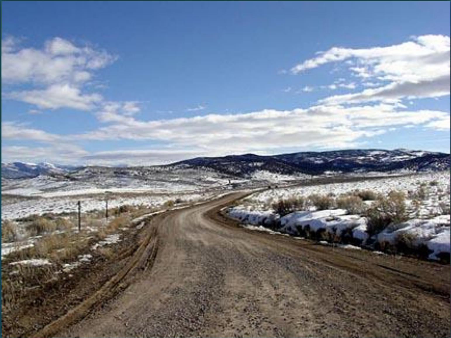
Road to The Property
